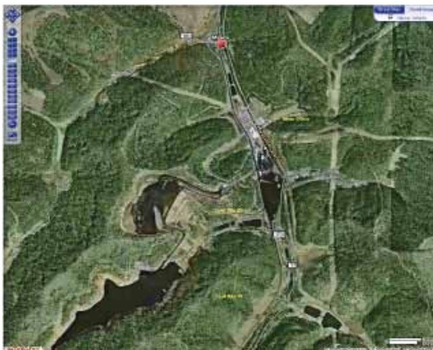
Figure 1. Aerial view of Federal mine #2, West Virginia, and the two seismic test sites.
