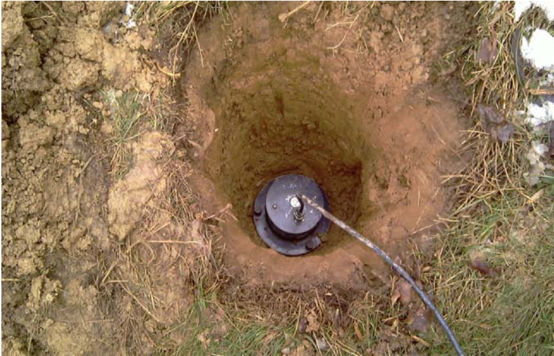
Figure 4. Photograph of surface sensor installation.
